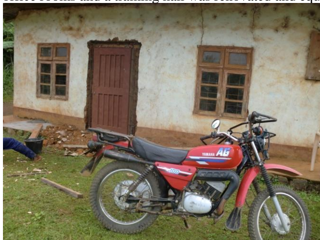
Office under Renovation
